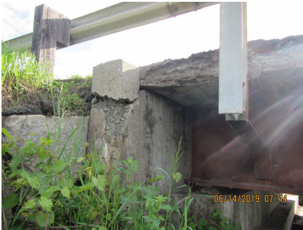
Picture 3: Fascia deterioration at backwall
