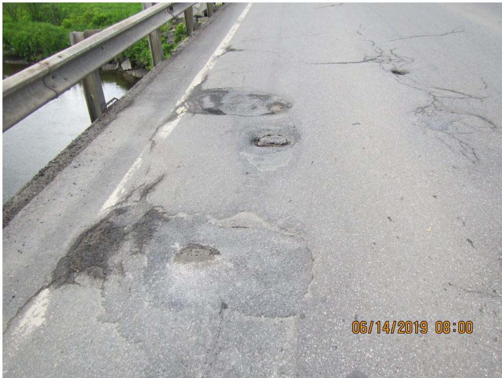
Picture 12: Potholes in wearing surface
