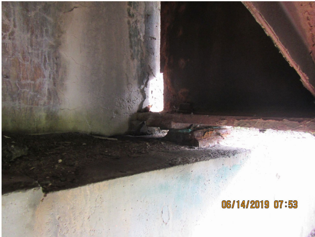
Picture 11: Section loss at beam end
