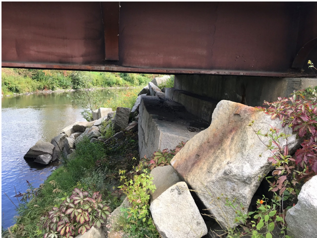
Figure 3.4: Facing southern abutment; note stacked stone facing and rip rap on adjacent embankments.
