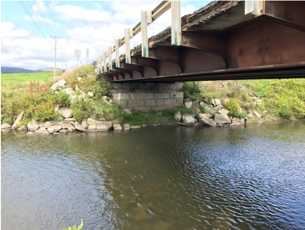
Figure 3.1: Facing northern abutment; note stacked stone facing and rip rap on adjacent embankments.
