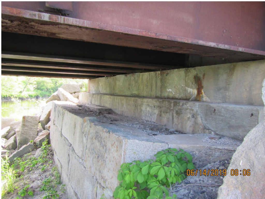
Picture 10: Bridge seat and abutment stem
