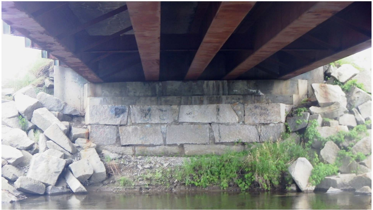
Figure 3: Substructure and abutments for bridge number 124.
