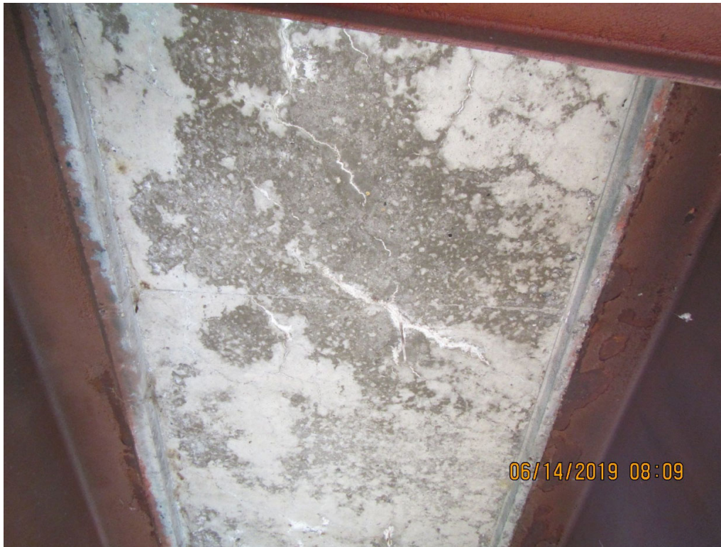
Picture 7: Saturation and cracking in deck
