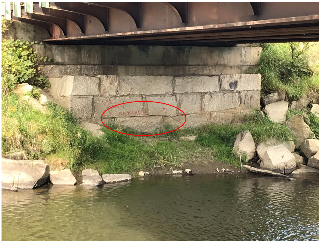
Figure 3.2: Facing northern abutment; note stacked stone facing and lack of mortar at some block connections (highlighted).
