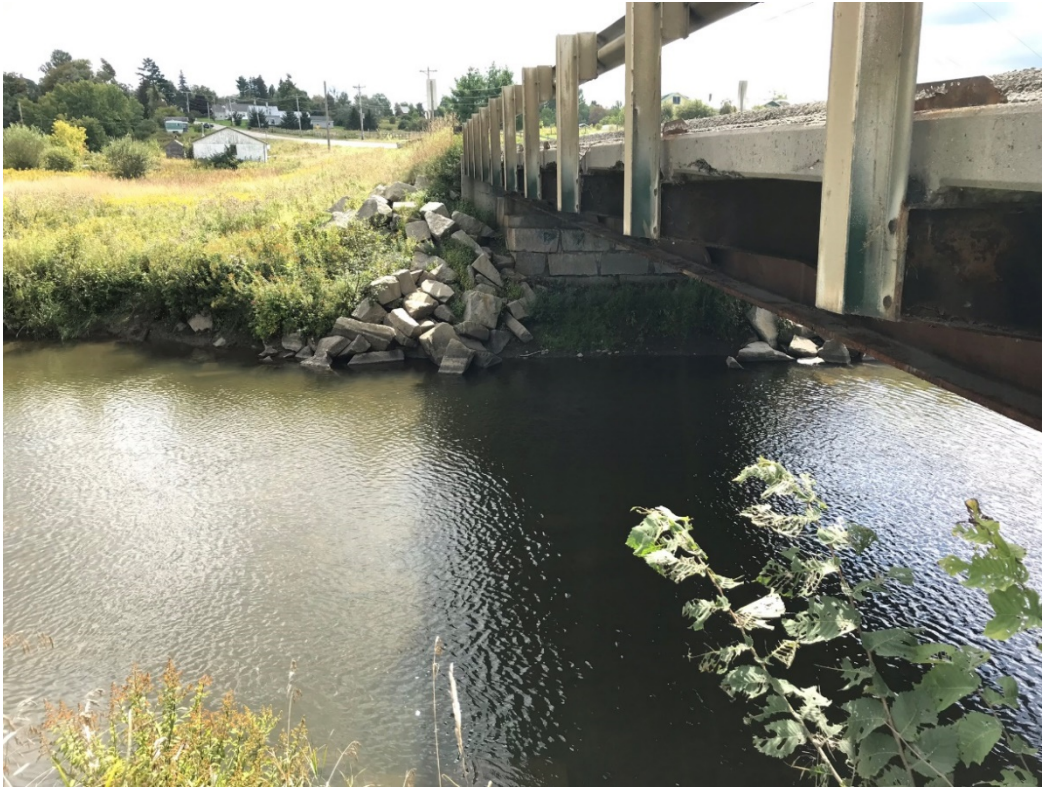
Figure 3.3: Facing southern abutment; note stacked stone facing and rip rap on adjacent embankments.
